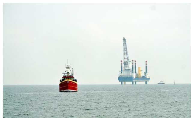
Installation vessel for offshore wind turbines with safety vessel (© BSH)
