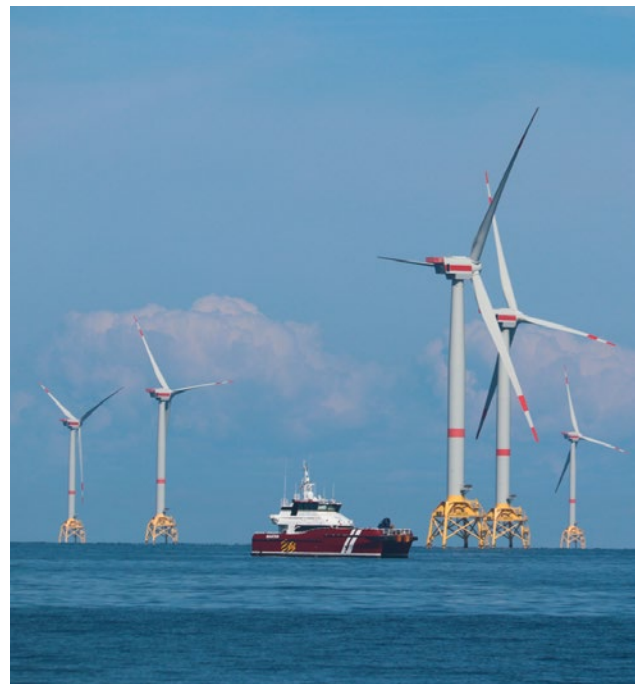
Offshore wind turbines in the Baltic Sea with service vessel
