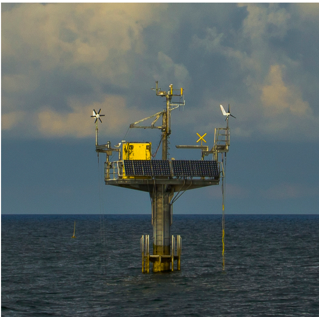
Measuring Station Arkona Becken (Photo: Mike Sommer, IOW)
