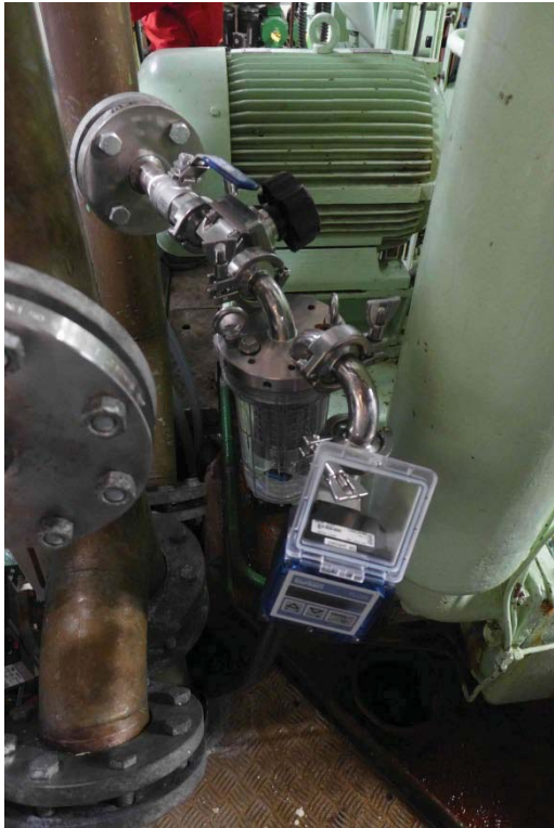
Figure D.3: Triton NP 6007 TG 18 skid: installation during hydraulic tests
