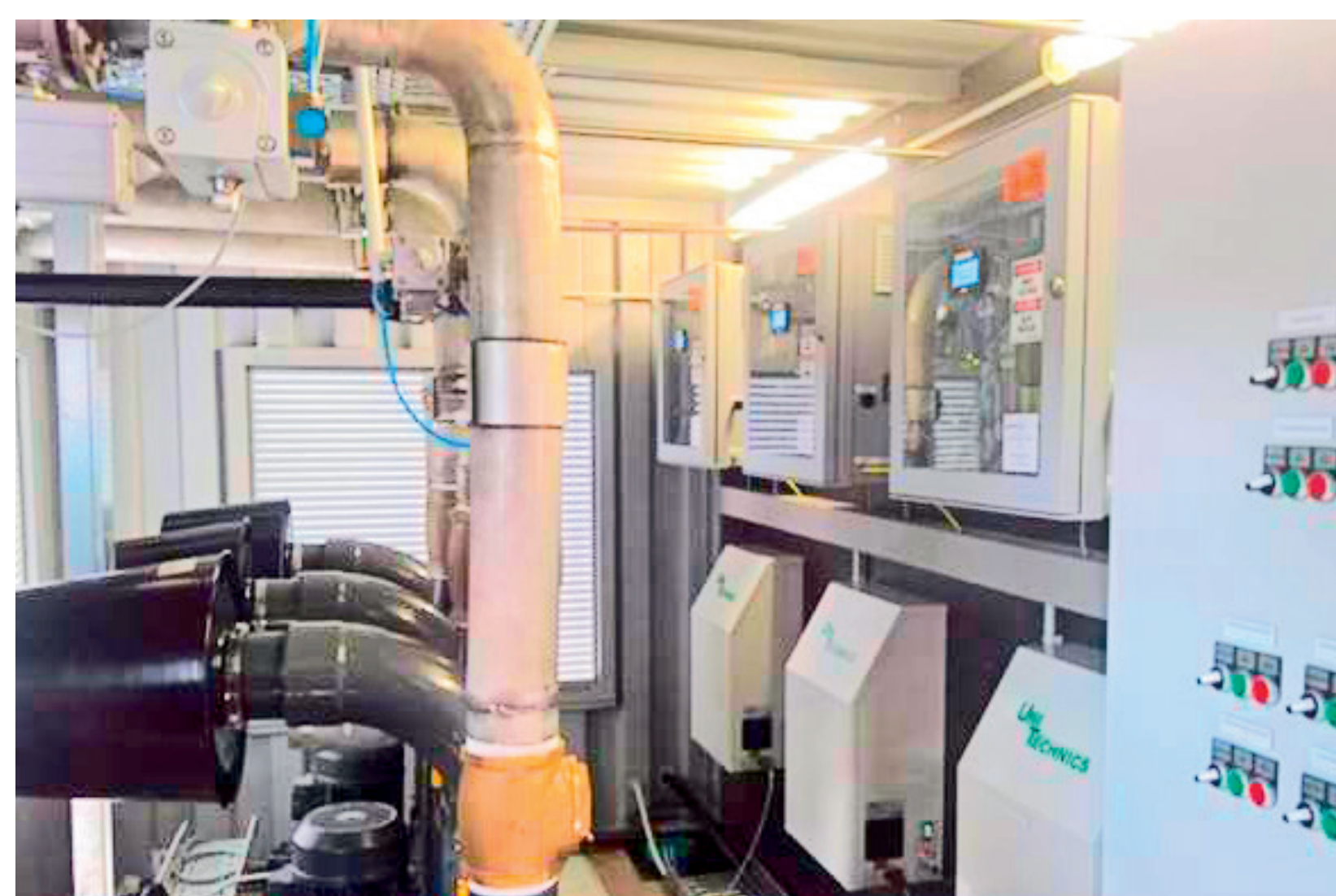
Solution at the Port of Kiel: PRF installation including analysis and pre-treatment for odor elimination and pH adjustment
