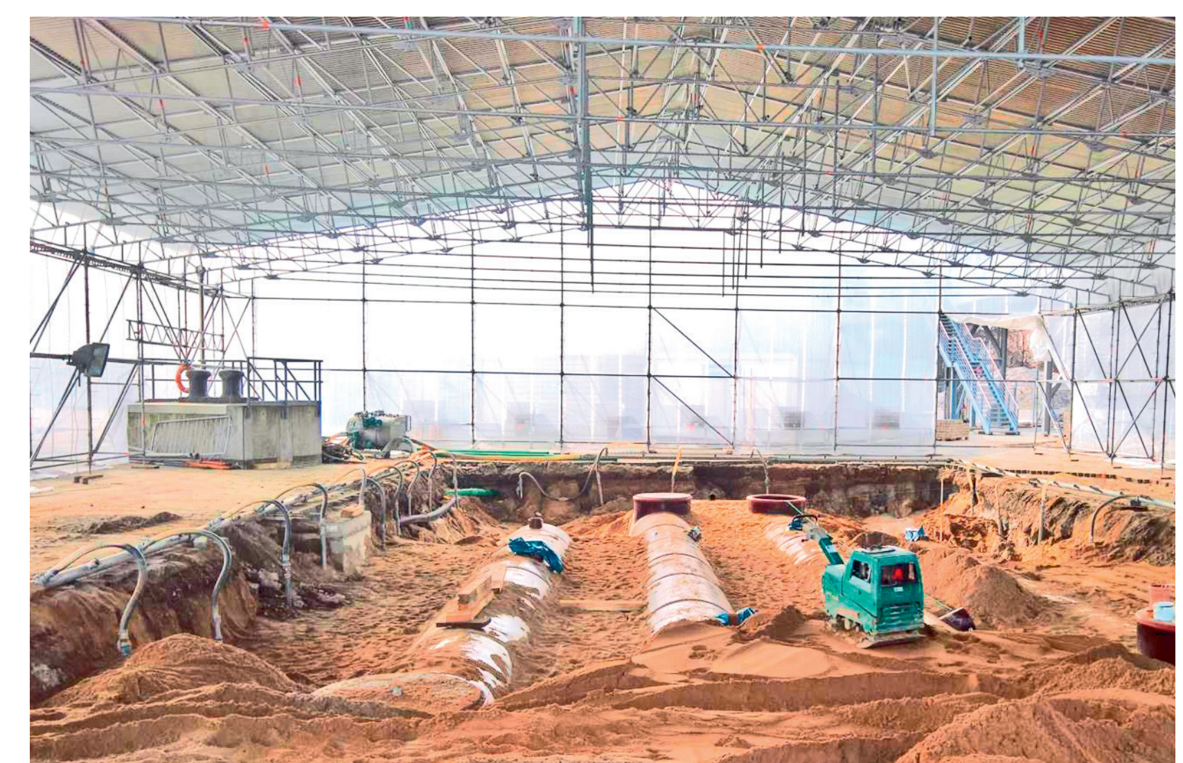
Solution at the Port of Kiel: PRF installation including analysis and pre-treatment for odor elimination and pH adjustment
